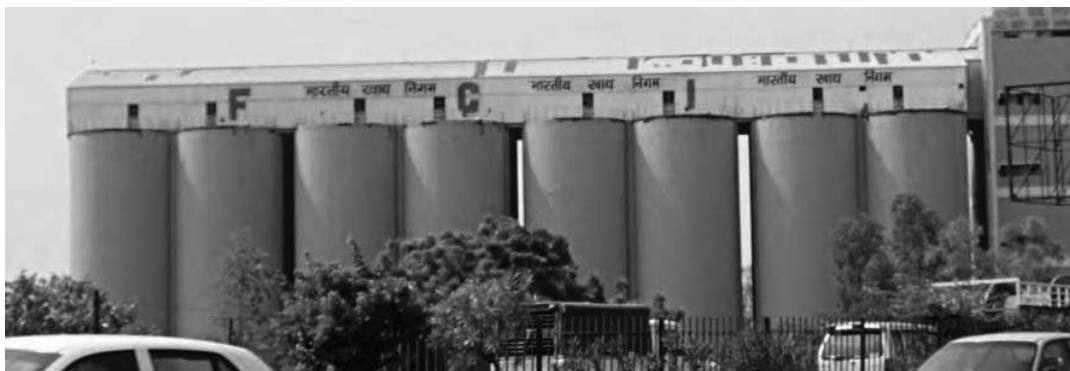
Fig. 1.10 (a) : Silos for storage of grains
