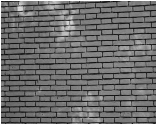
(a) Brick wall
