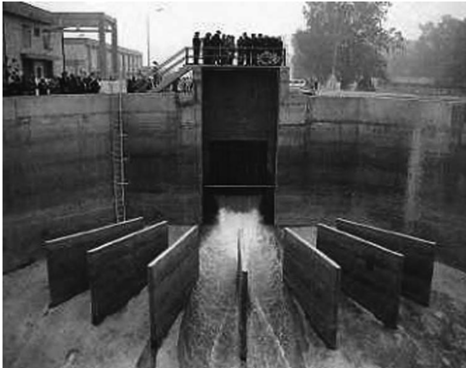
Fig. 18.10 : Water treatment plant
