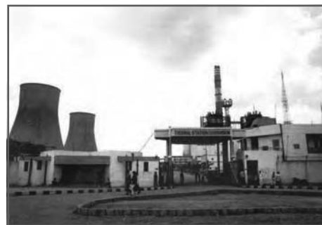
Fig 3.12: A view of a Thermal Power Station
