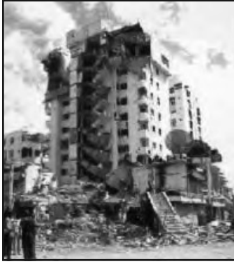
Fig. 3.3a: Destruction caused by an Earthquake at Bhuj
